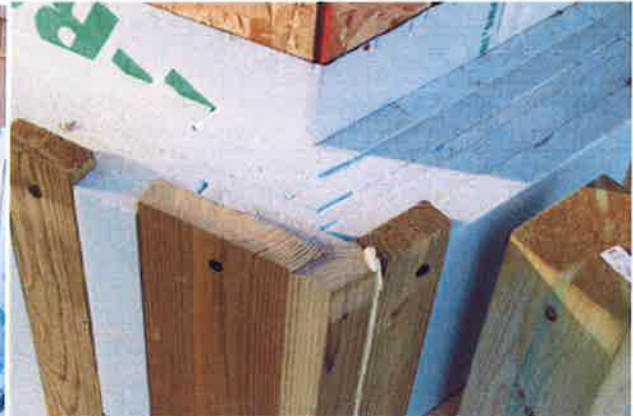
A three inch correction was made on the north wall and a nine inch correction was made on the west wall to correct previous construction errors. Six inches of XPS was added to all basement walls.
