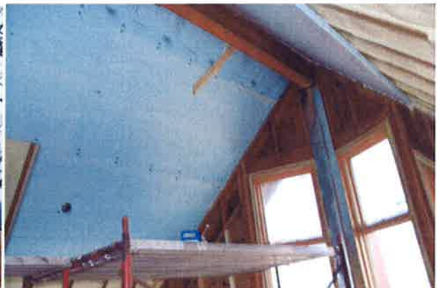
PIC insulation which has lower imbedded energy was used on all other exteriors walls and for interior foamed surfaces. One inch of rigid foam was added to provide a thermal break on the ceiling.
