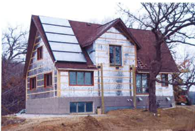
PIC insulation which has lower imbedded energy was used on all other exteriors walls and for interior foamed surfaces. One inch of rigid foam was added to provide a thermal break on the ceiling.
