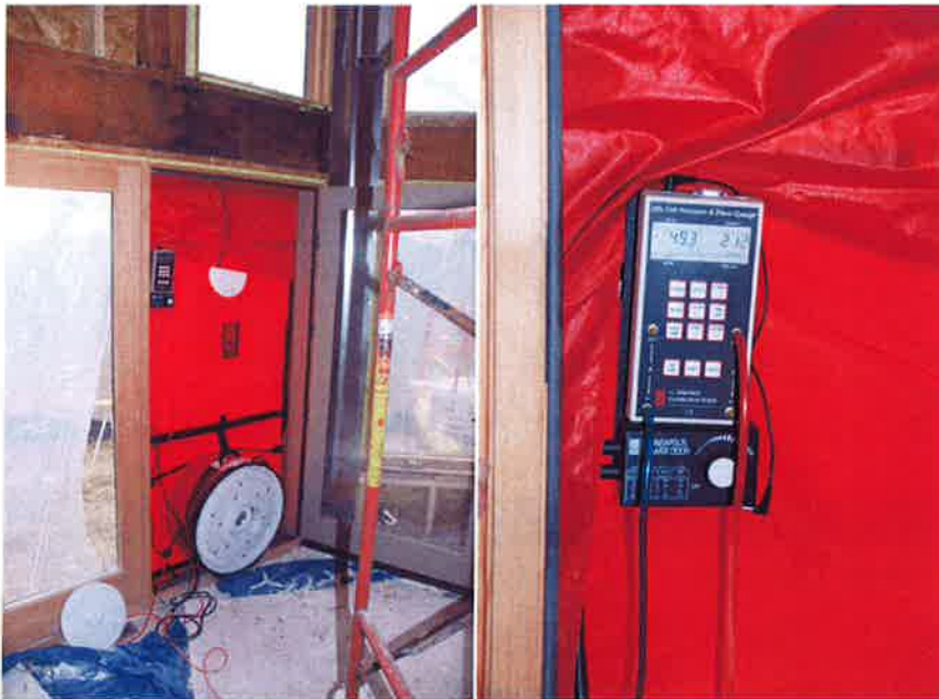
Blower door test were used to verify air tightness. Air tightness went from over 6+ Air Changes per Hour (ACH) at 50 Pascal's of pressure to 0.45 ACH, >92% improvement.
