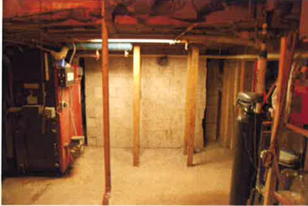
Old wood burning furnace in basement which used @ 17 cords of split, dried oak firewood a year and the new solar thermal system utilizes the in-place hydronic heating system.
