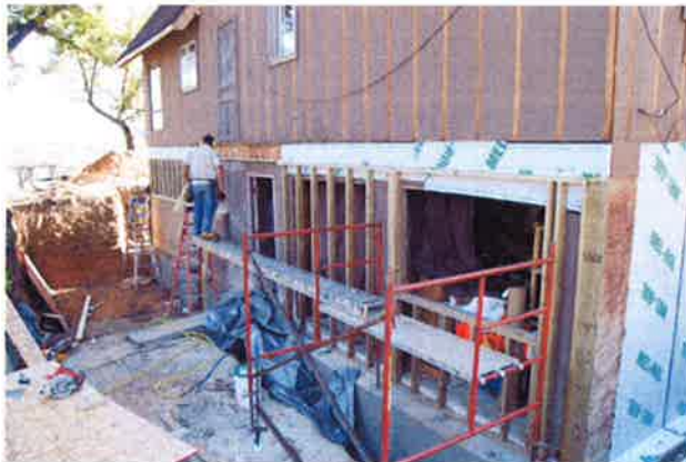
A three inch correction was made on the north wall and a nine inch correction was made on the west wall to correct previous construction errors. Six inches of XPS was added to all basement walls.
